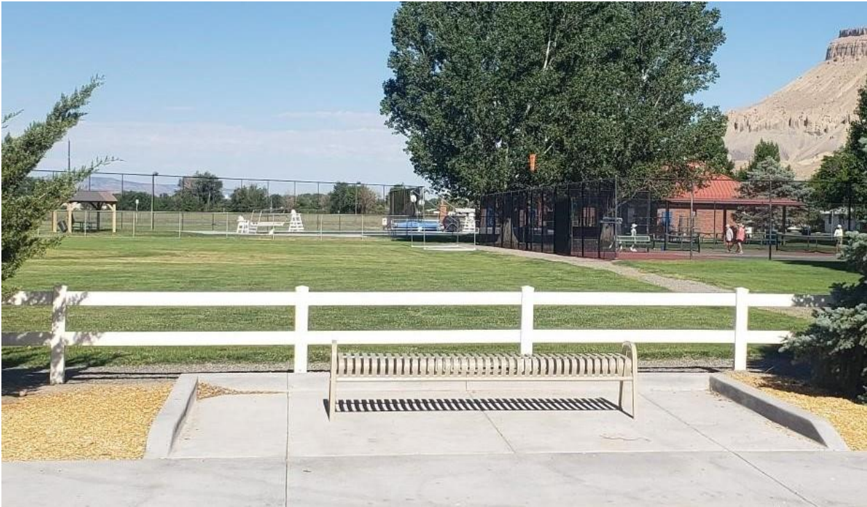
New bench installed at Peach Bowl Park with completed grading and mulch.
